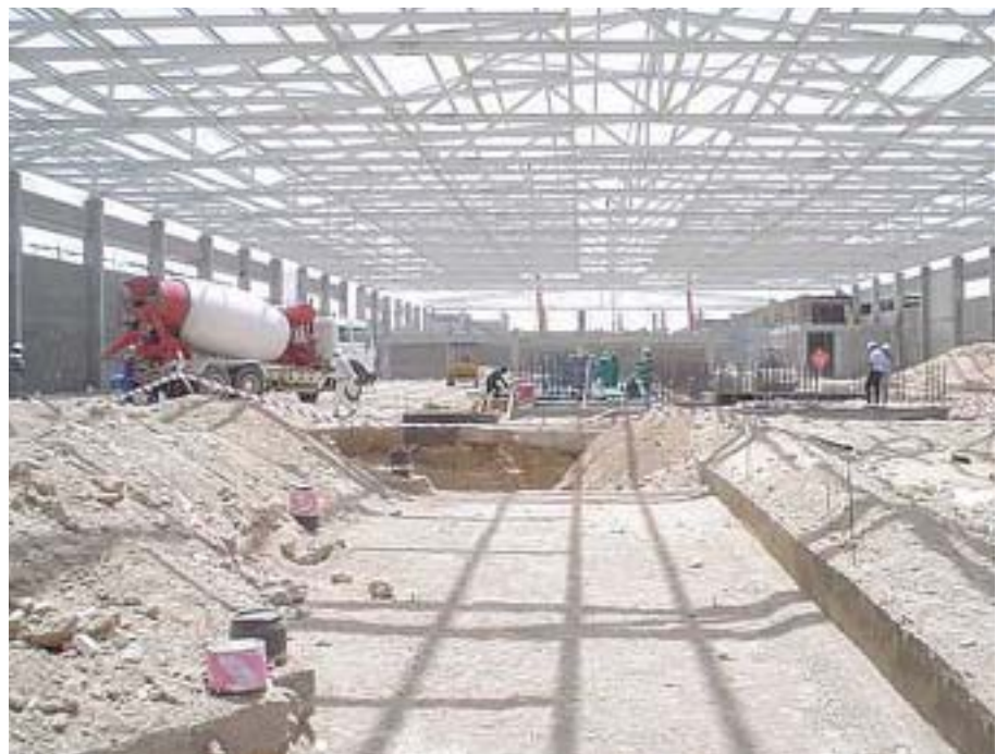
Looking down the 185m factory length from what will be the wet end towards the finishing department. Excavations in the foreground are for segregated drainage for different process outflows and the reinforcing (centre) is the start of the mezzanine floor for drum processing.
